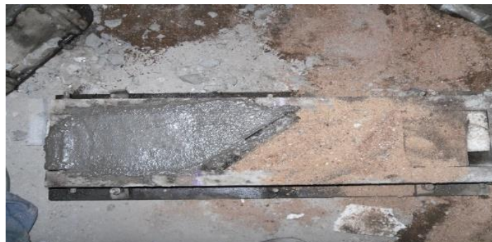
Figure 7. Casting of new substrate with steel plate creating an angle 45 0
